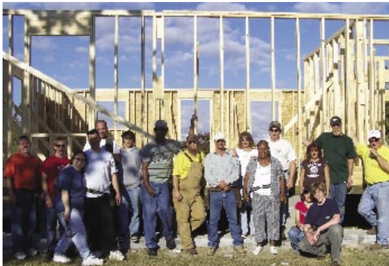
Members from Hillcrest Covenant Church and Castle Oaks Covenant Church (Colorado) join residents of Phoenix in rebuilding homes destroyed by Katrina.
