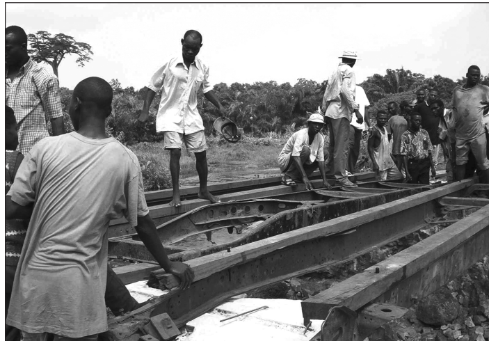
Covenant World Mission and the Paul Carlson Partnership are working on rebuilding bridges in northwestern Congo.
