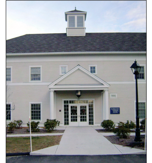
With its distinctive cupola, the new two-story Family Treatment Center at Covenant Children’s Home of Cromwell reflects features of the original tabernacle that was an icon on the hilltop campus.
