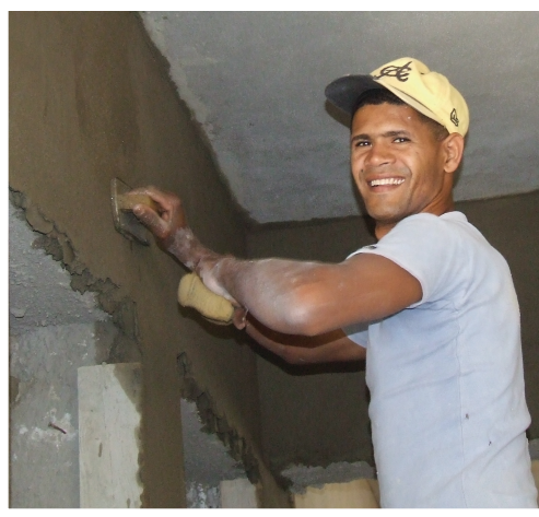
A mission team member works on a wall.
