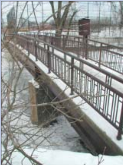
The bridge where the homeless man's body was found. Beyond the bridge North Park's athletic field can be seen.
