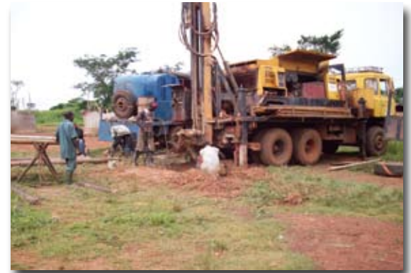
Potable water and electricity are needed
