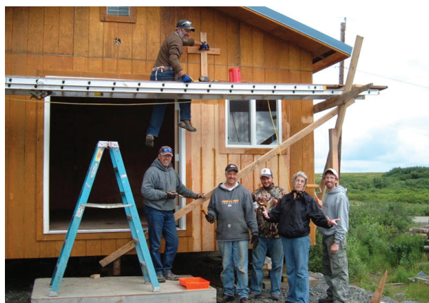
Putting the finishing touches on a utility building in Mountain Village—team members came from at least four different churches in the Midwest Conference.
