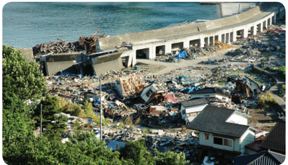
Destruction following the devastating earthquake and tsunamis in Japan.
