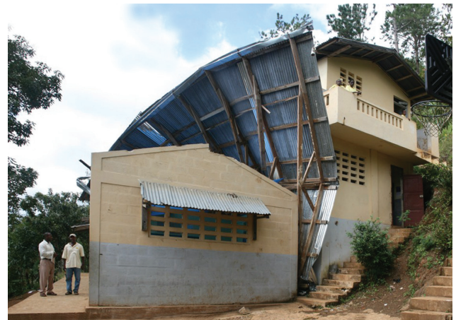
The first room of the school was built with the help of North Park students (top left). Construction continued on a second building behind the first (top). Hurricane Sandy tore the roof off the original building (above).
