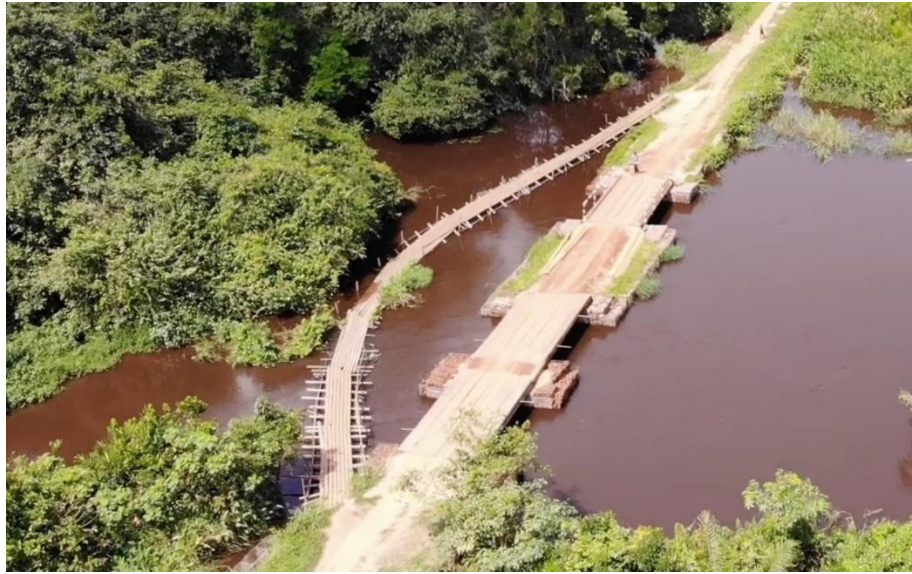
Completed bridges (walkway will be removed)
