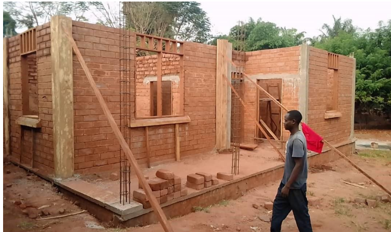
Malnutrition Stabilization Center under construction in Karawa
