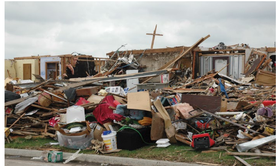
Devastation after Moore, OK tornado.
